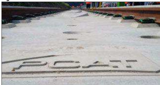
Figure 6: The test line of the PCAT system
