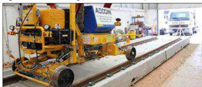
Figure 7: The RTST testing (AECOM PCAT Test report)
