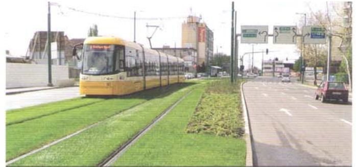
Szeged, line II; inductive loop built in EPC fibre-reinforced concrete structural plate, grassy track section
