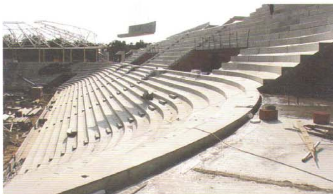
Debrecen's Nagyerdei Stadium, prestressed Barchip 48 synthetic fibre-reinforced concrete grandstand elements
